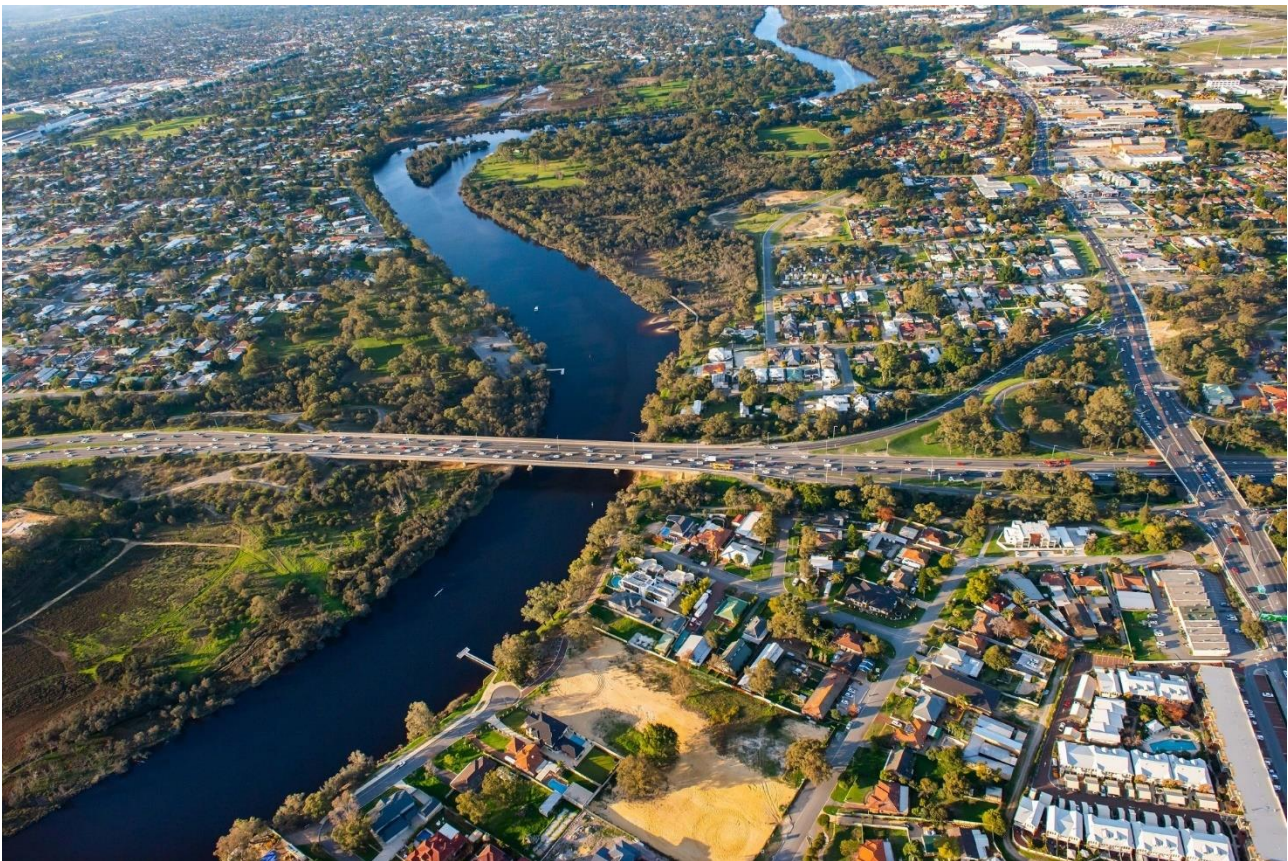
Figure 20 Redcliffe Bridge linking the cities of Bayswater and Belmont via Tonkin Highway (over the Derbarl Yerrigan)
