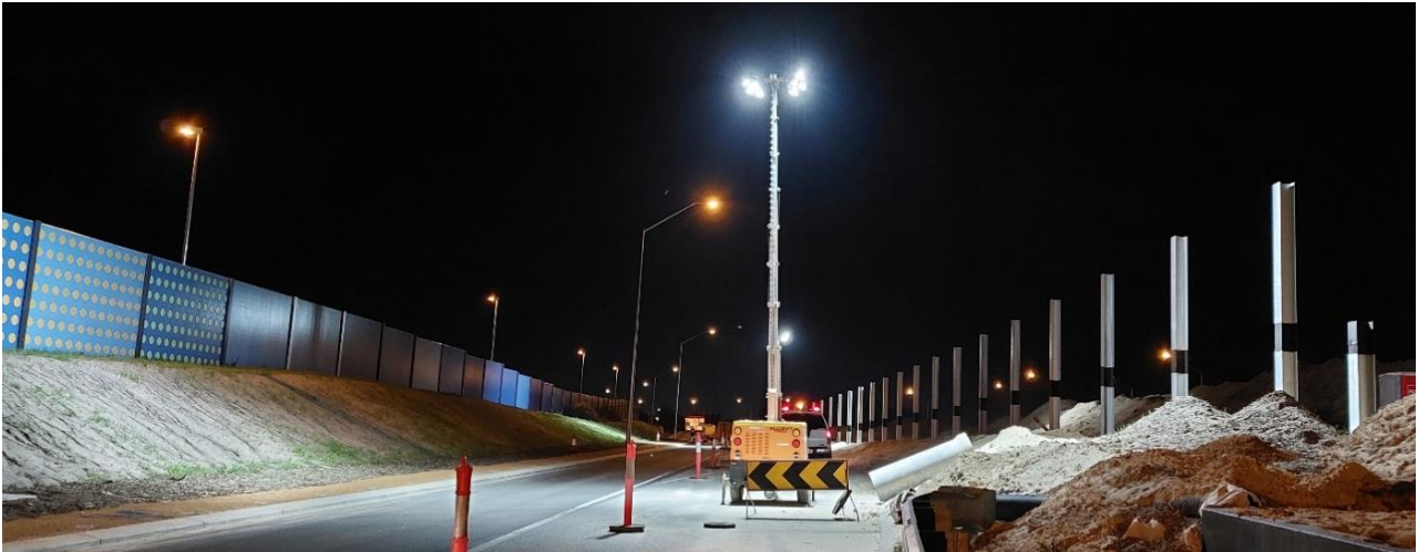
Figure 16 Light tower used during nightworks
