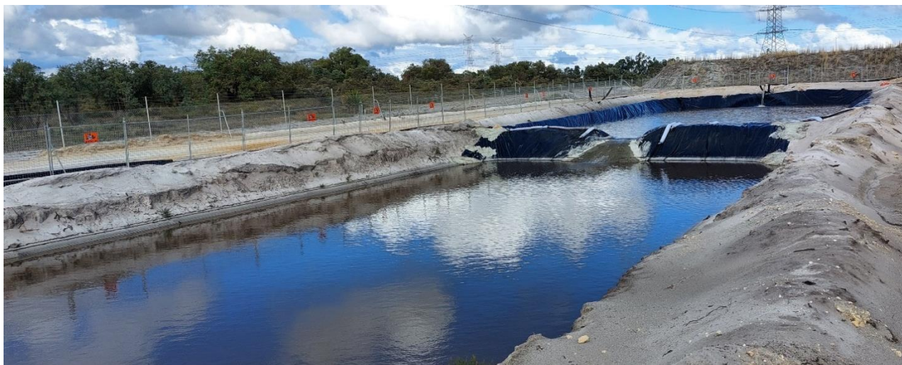
Figure 13 Main infiltration basin located at the northern dive structure
