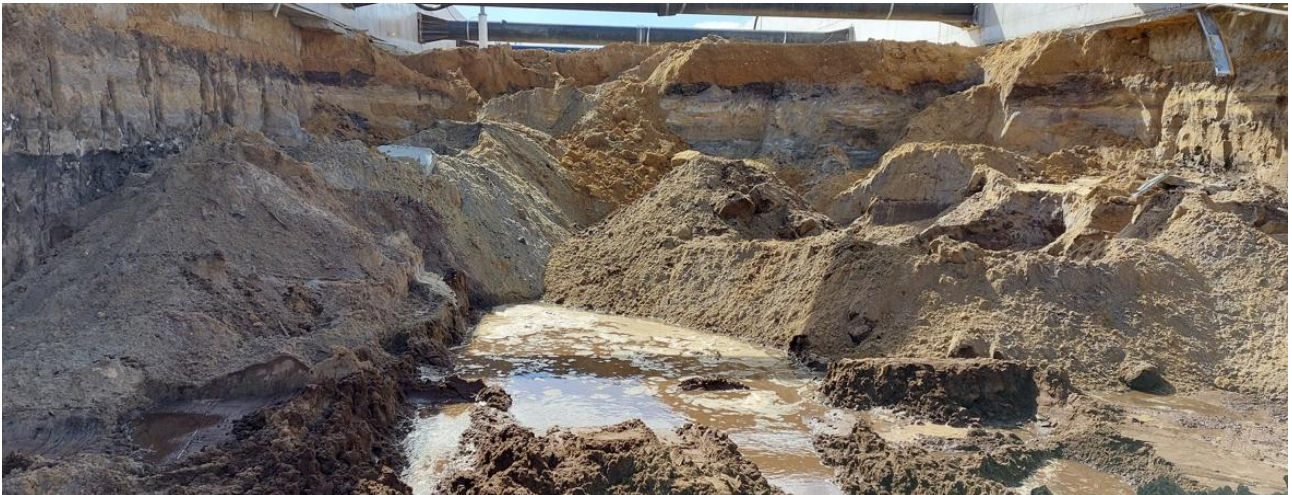
Figure 18 Bulk excavation at the northern dive structure
