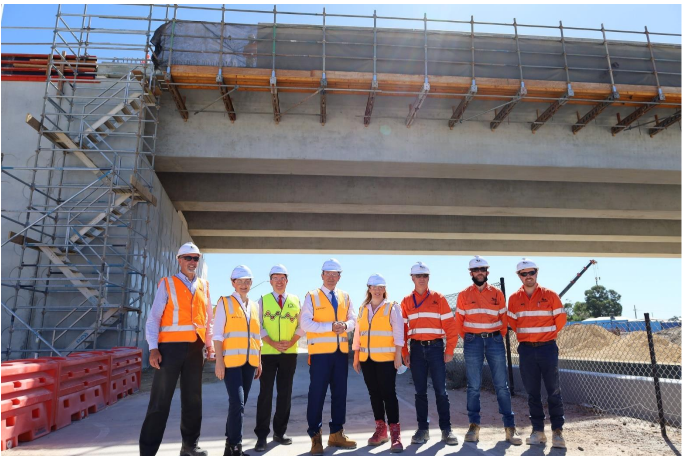
Figure 10 Broun Ave Bridge deconstruction tour with Premier Mark McGowan, Transport Minister Rita Saffioti, Health Minister Amber-Jade Sanderson, Water Minister Dave Kelly and Main Roads and TGA representatives.
